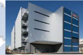
Industrial Mechatronics Systems Works/ Nagoya Works
